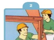
2 To prop up metal door frame, use two planks with nails at the ends. Ensure the correct direction of your door hinge then erect the door frame. The nails on the plank should hook to the edge of the frame.
