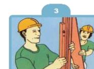
3 To check whether the frame is properly plumbed, use a spirit leveler.
